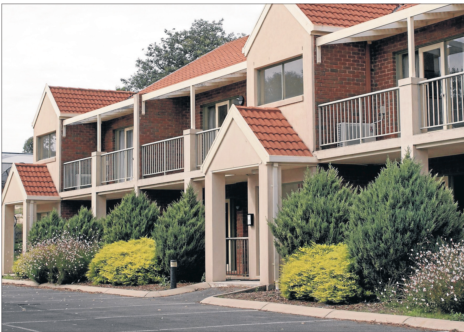
AUCTION: The Ballarat Colonial Motor Inn will be auctioned later this week.
